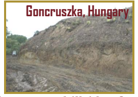
↑ Steep hillside of cemetery deteriorating
